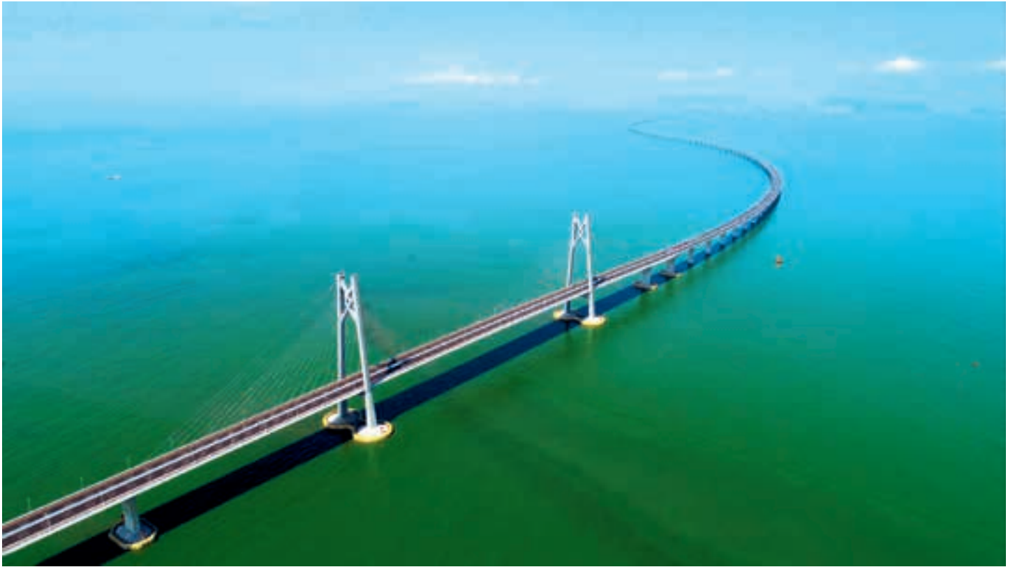
The Hong Kong-Zhuhai-Macao Bridge, which is the world largest ever sea-crossing project with a total length of 55 kilometers
